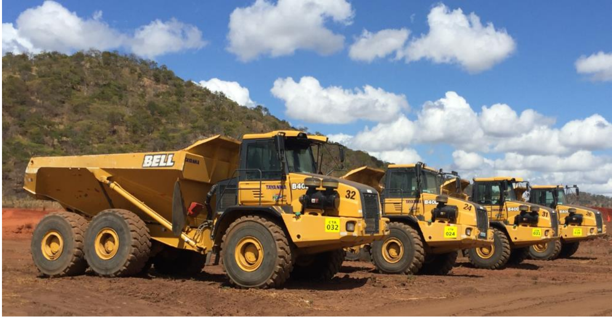
Figure 9 – Mining fleet mobilised on site
