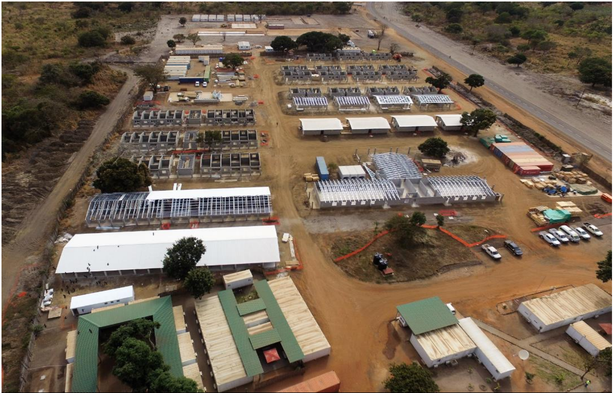
Figure 8 – Construction underway for the expansion of the accommodation camp
