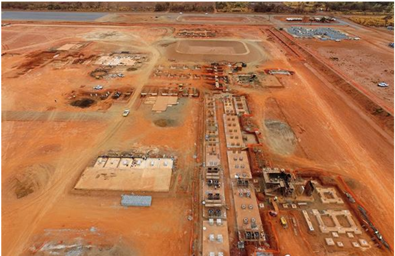
Figure 4 – Concrete foundations for the flotation circuit
