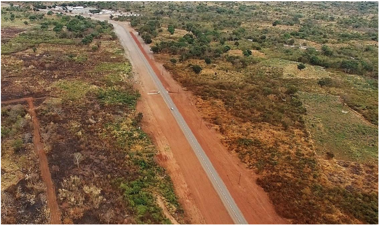
Figure 3 – Fully bitumised access road
