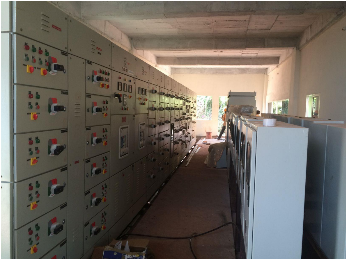
Internal Control Room Testing
