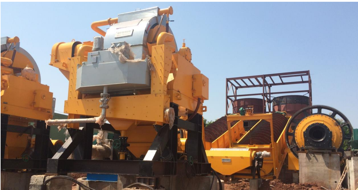
Final Fitout of Chinese Equipment
