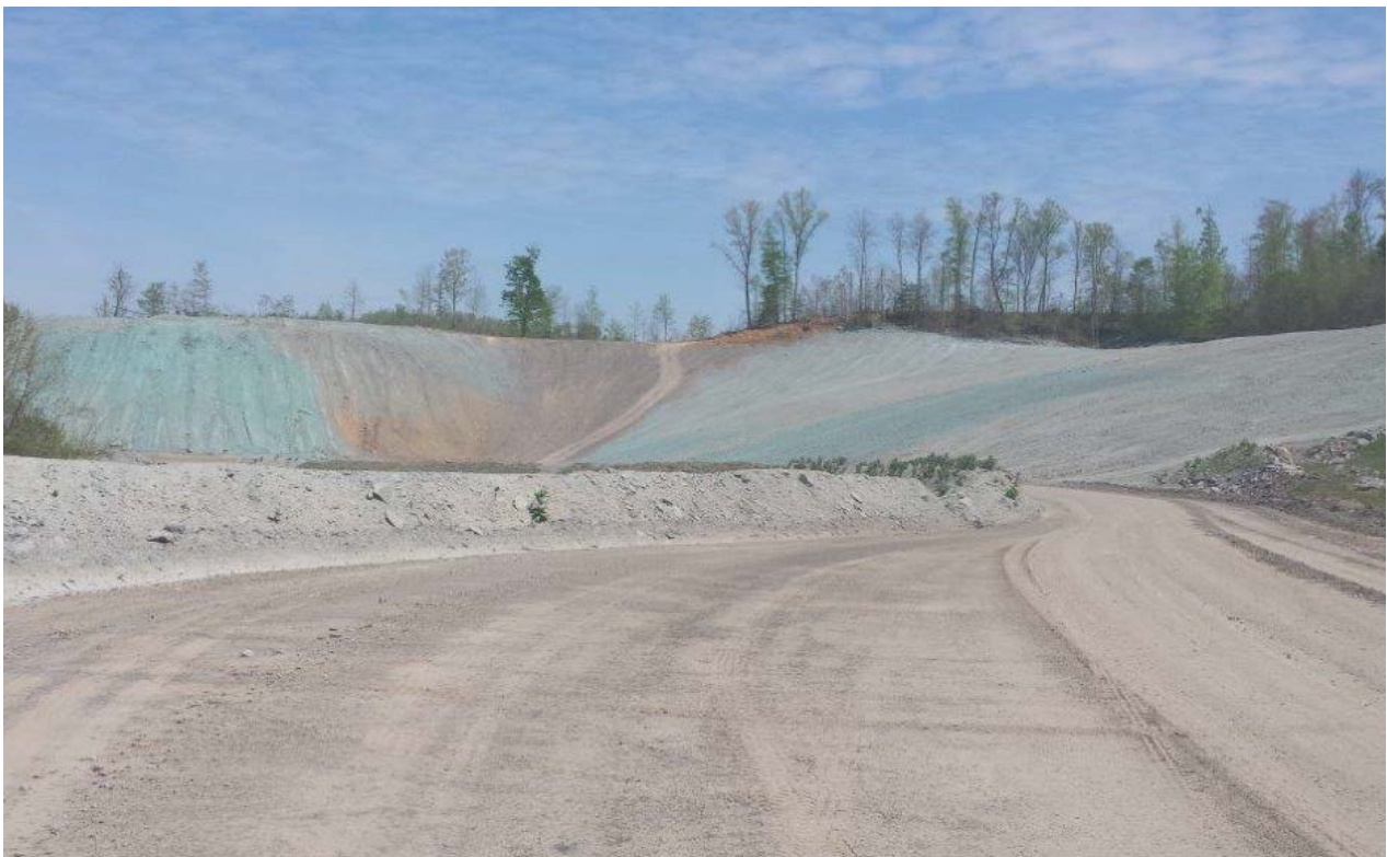
Reclamation Hydro Seeding at Flat Creek- Mountainside Coal Company Inc., Kentucky
