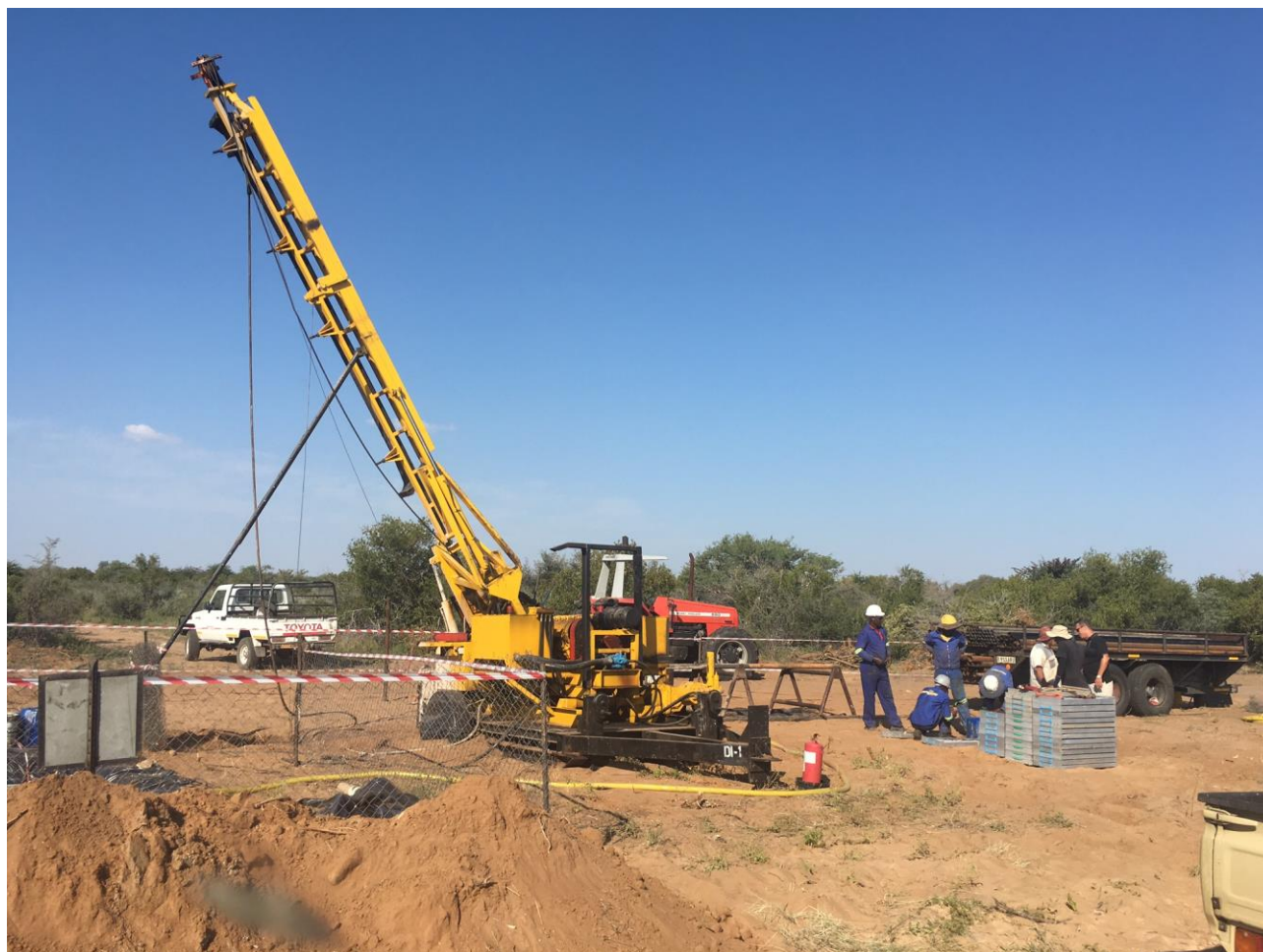
Figure 3: Diamond Drill rig at T3
