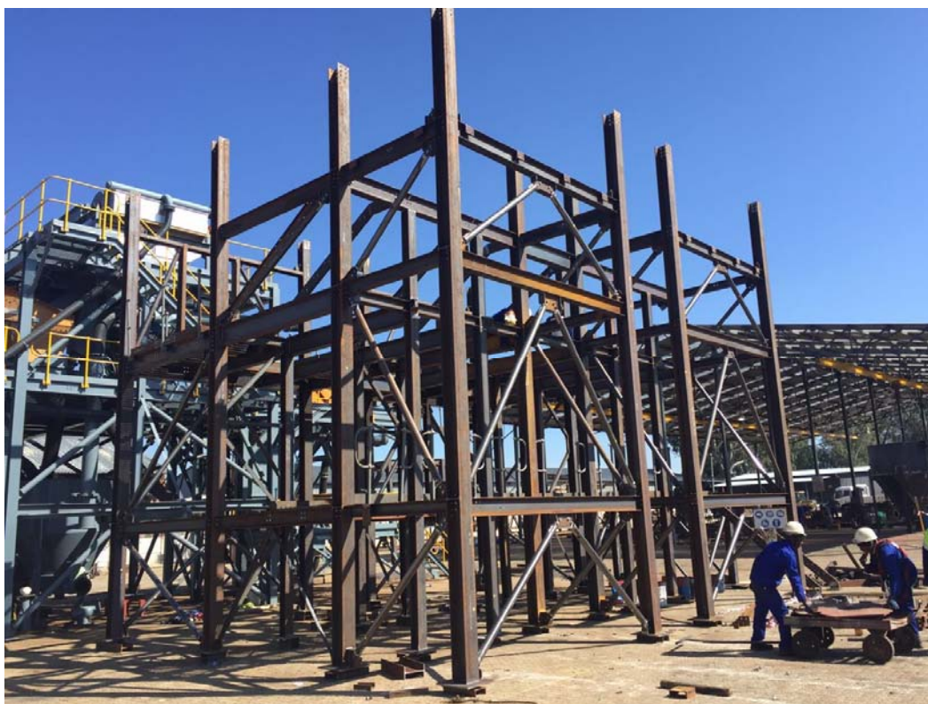
Figure 6: Offsite Trial erection of Process Plant
