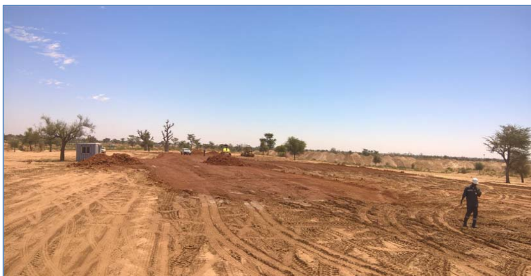
Figure 8: Preparation of the Process Plant area underway incorporating compacted laterite
