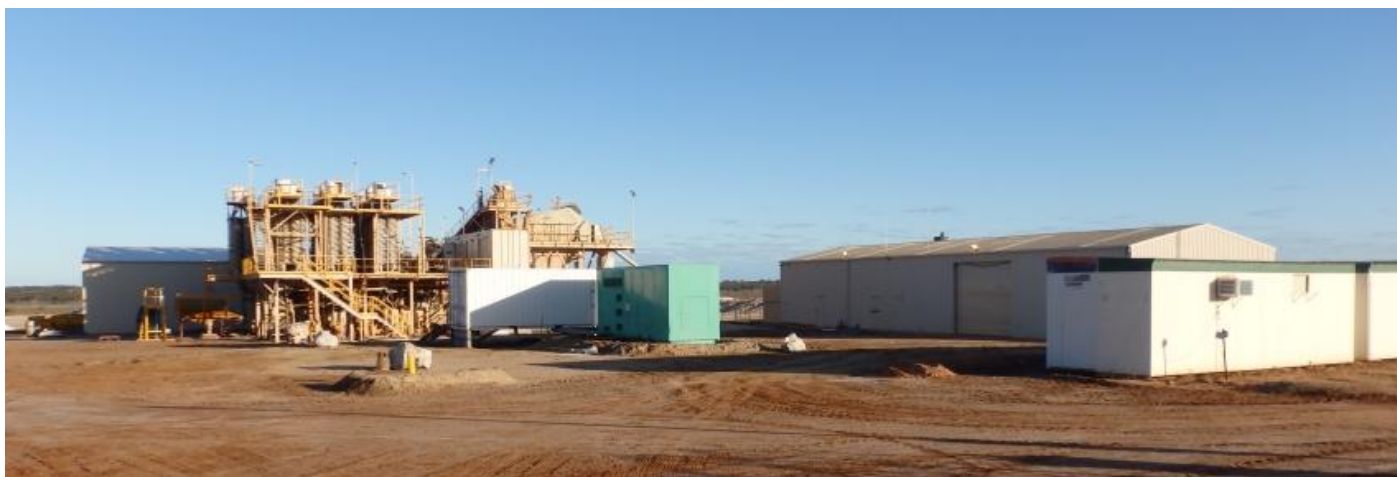
Overview of Tantalum Processing Facility - Bald Hill
