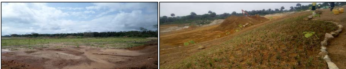
Figure 3. Rehabilitated mine block (at left) and slope-stabilisation planting to prevent run-off - Golu Mine.
