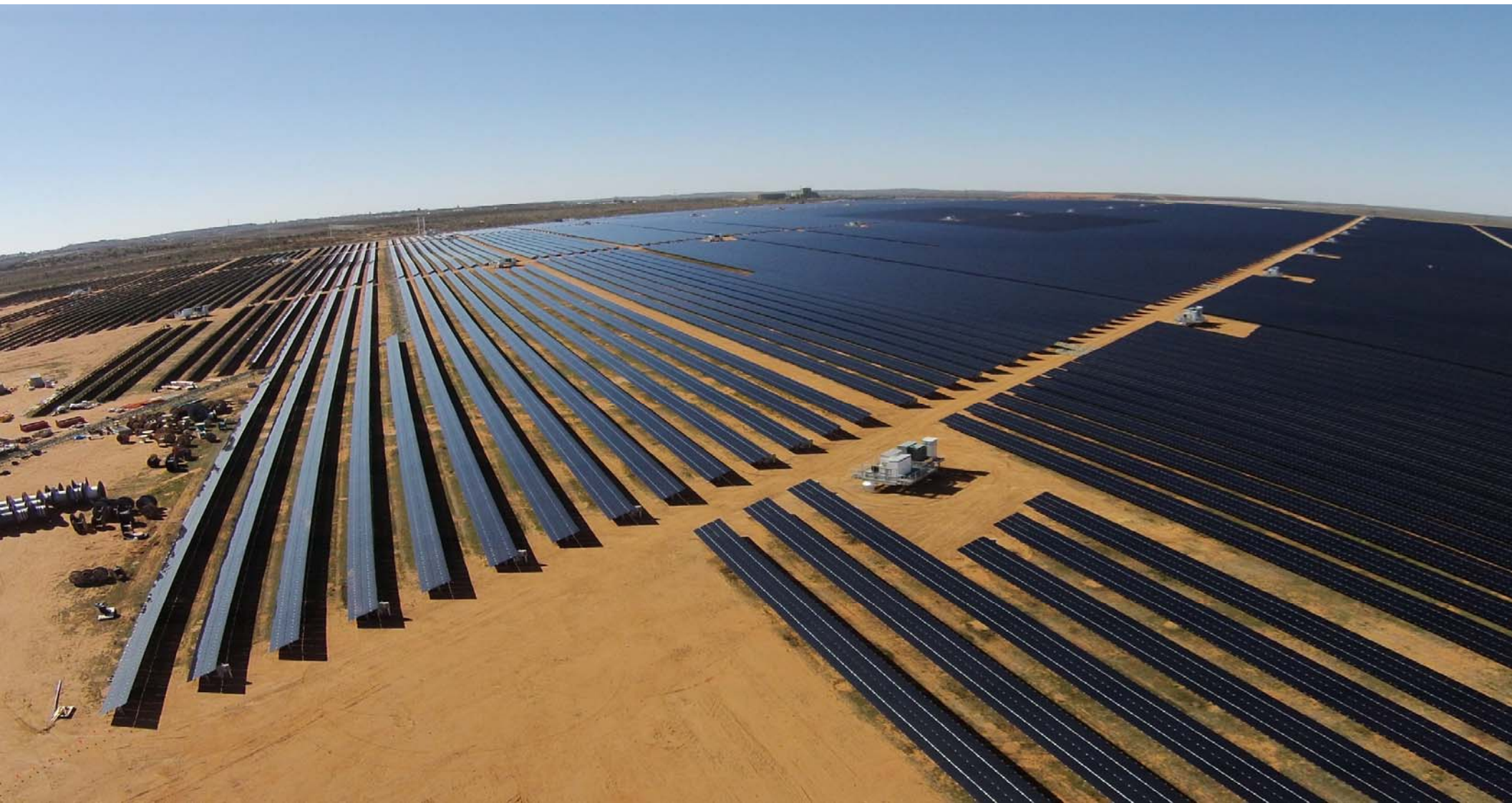
RCR completed E&I, installation and energisation of 680,000 Photo-Voltaic panels for AGL's 53MW Broken Hill Solar Project, NSW
