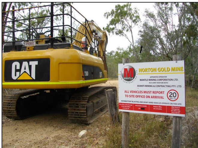
Picture 1: Mobilising to site.
