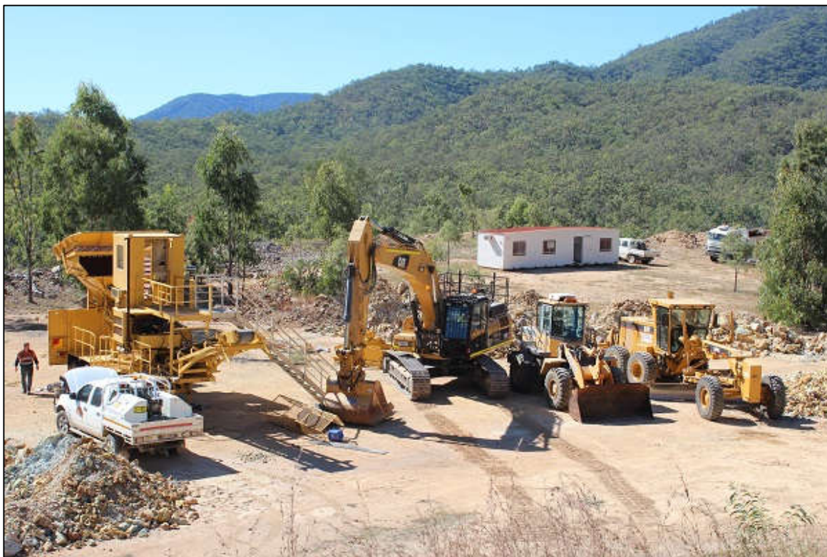
Picture 3: Site earthmoving and crushing fleet at Frampton stockpiles.
