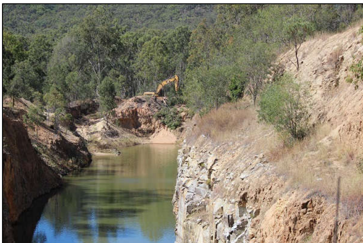
Picture 2: Excavating Never Never shear.
