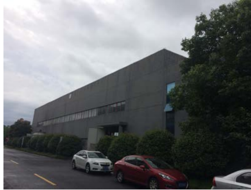
Picture of the leased premises in Changzhou Industrial Park
