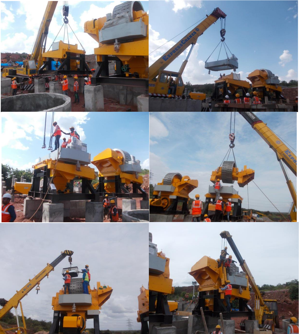
WHIMS Number Two Erection
