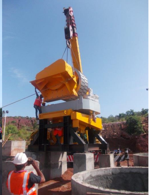
WHIMS Number One Erection
