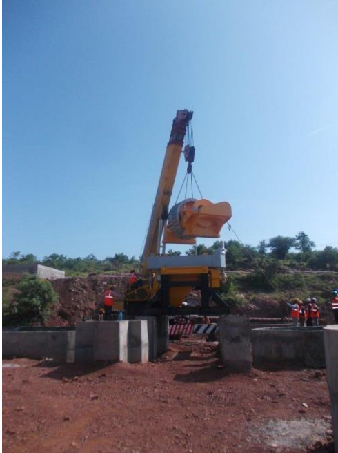
WHIMS Number One Erection
