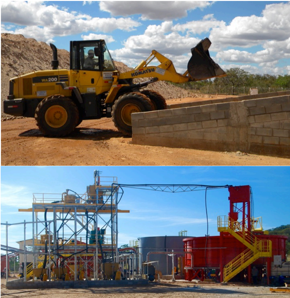
Top: Front-end loader reversing down the ramp to the grizzly with a stockpile of ~6kt of low grade commissioning material in the background. Bottom: Gravity tower and thickener with process water tank in background.
