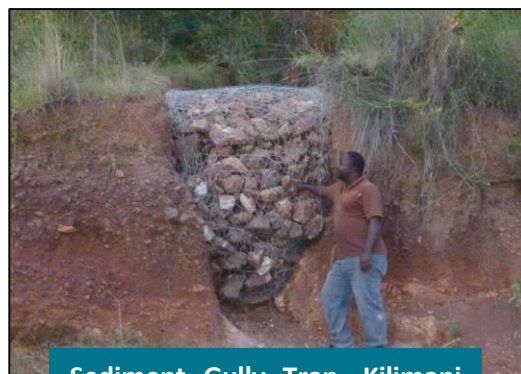
Sediment Gully Trap, Kilimani
