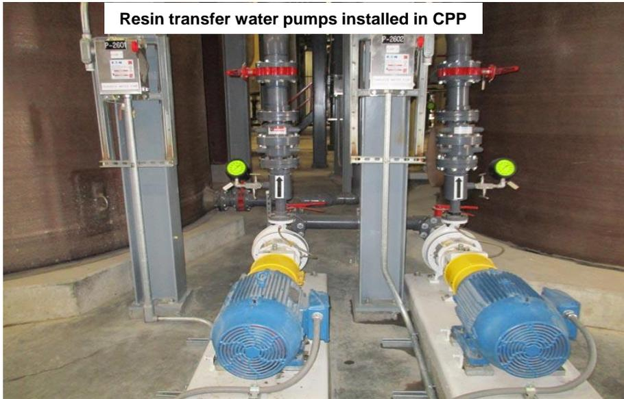
Resin transfer water pumps installed in CPP
