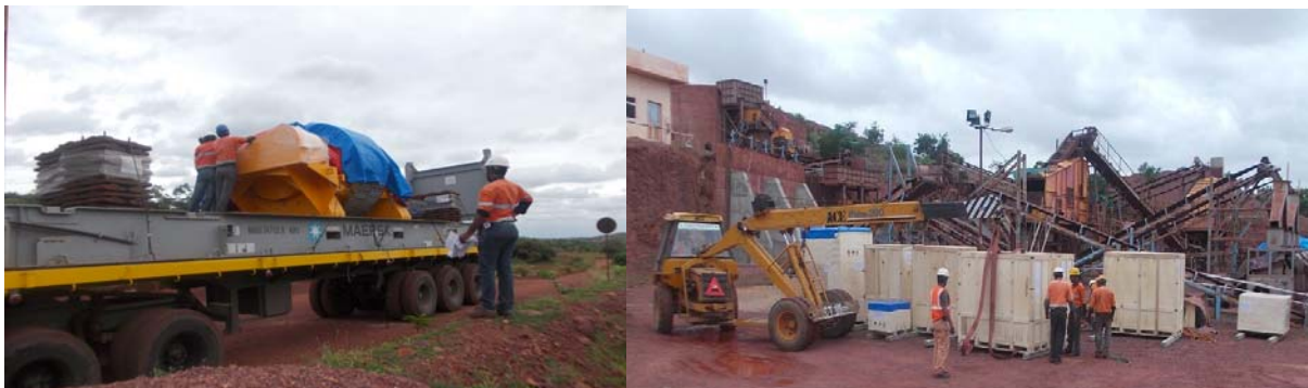
Further equipment unloading at site
