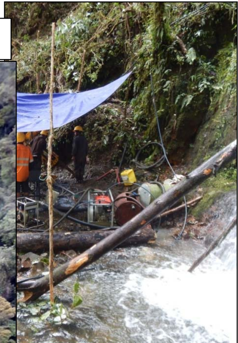
Hole EZU001 drilling 40° incl. to right, collar in front of RH Offsider. Target is 2.0m grading 195 g/t. View to NW is slightly skew of gold zone
