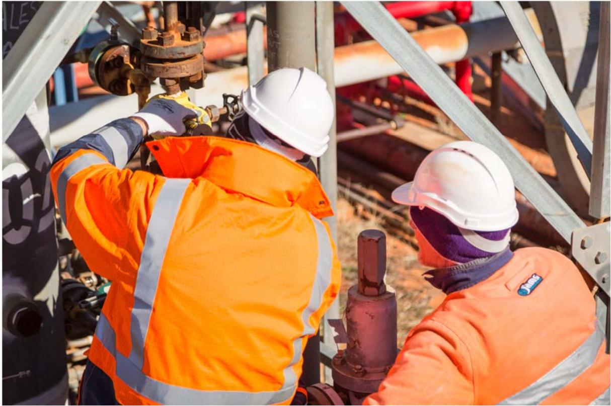
Figure 4: Mereenie; Maintenance at Central Treating Facility.
