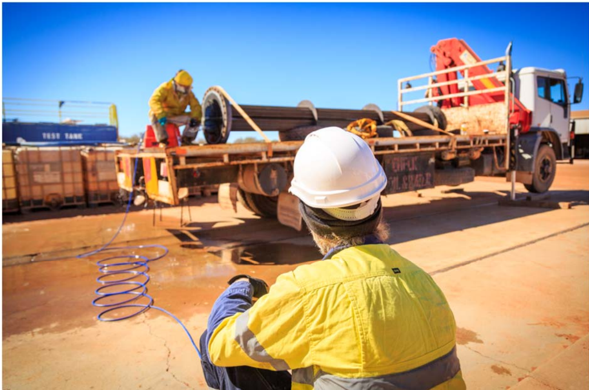
Figure 5: Cleaning Heat Exchanger Core.
