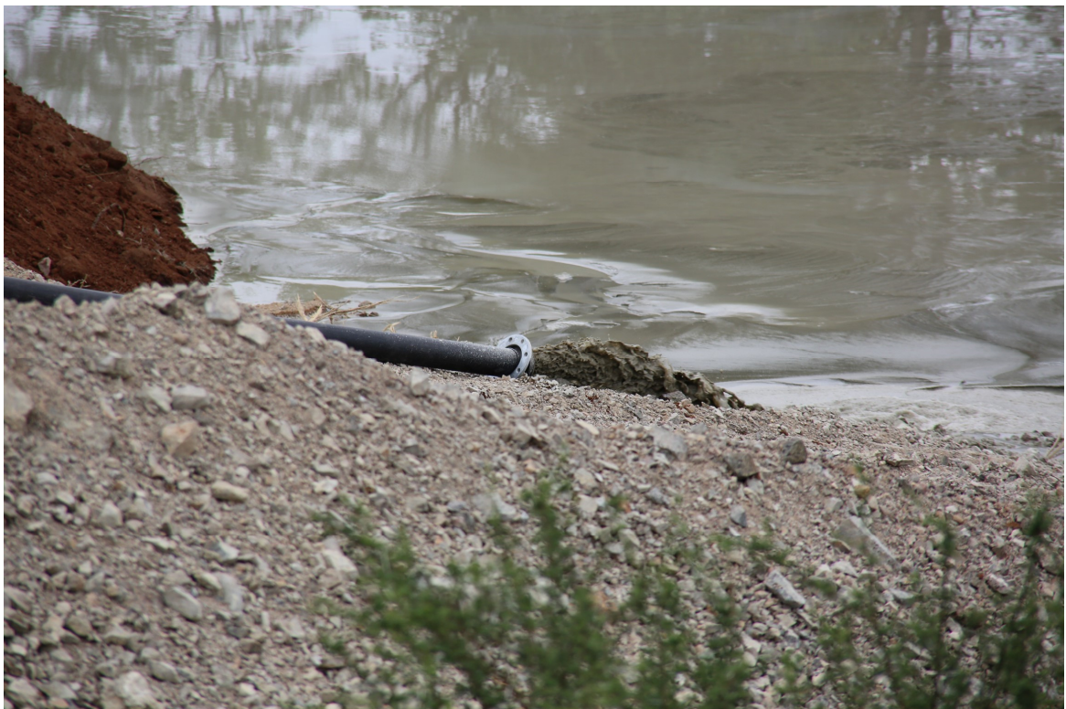
The first wet tailings being pumped into the slimes dam
