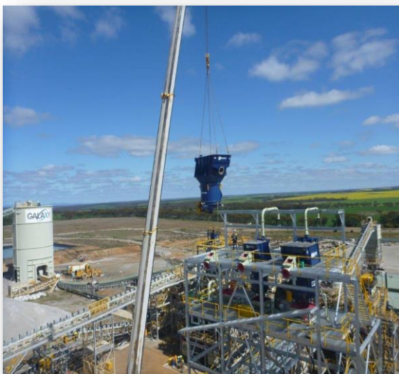
Lifting Final Reflux Classifier into Position
