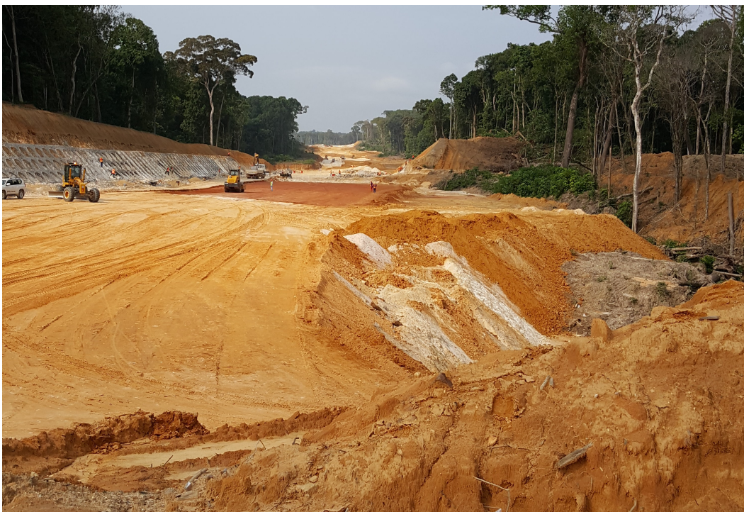
Figure 4: Earth works at the Kribi Port area for the new highway and rail
