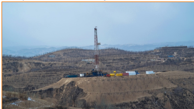
Third Party Drilling Rig
