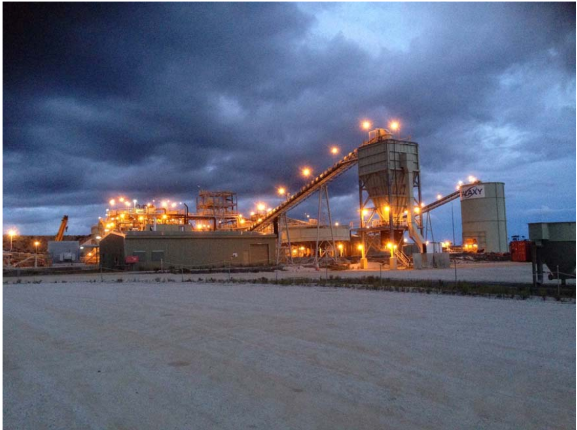
Figure 1 Mt Cattlin plant
