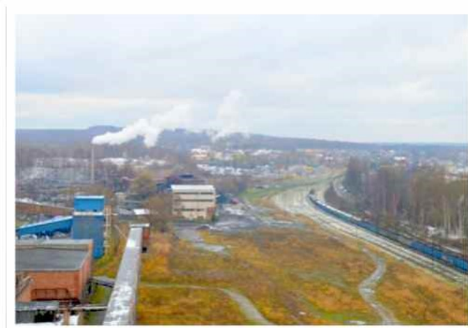
Figure 3 – Existing Site Facilities
