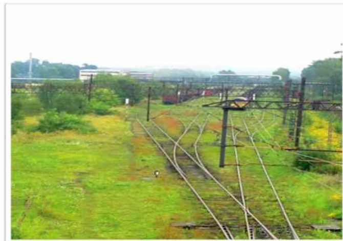
Figure 4 – Railway Siding at Debiensko
