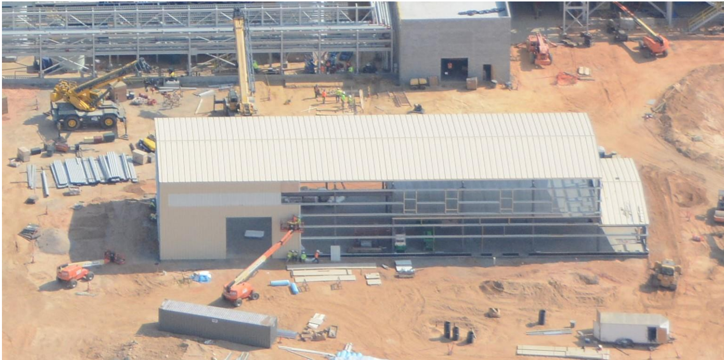
Area 940 Mill Maintenance Building
