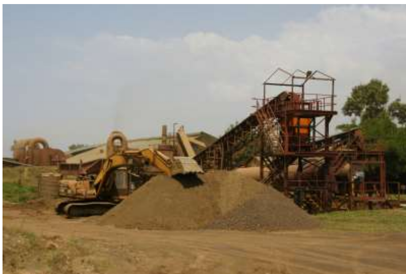
Photo 7: The Plant Crushing and Screening Operations Located on ML4651
