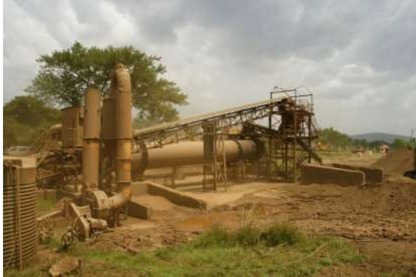
Photo 11: View of Plant Showing Blowers and Heating Furnaces Located on ML4651
