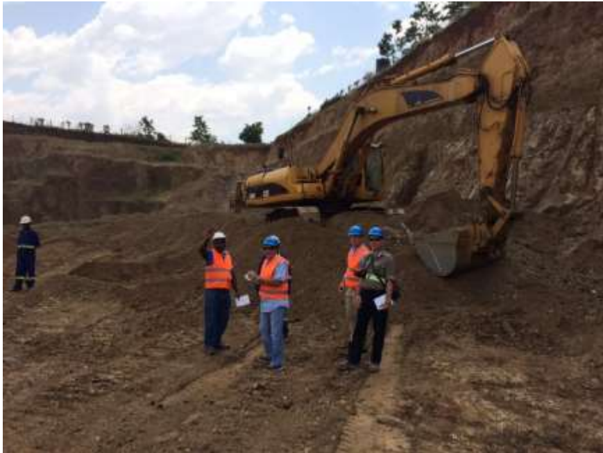
Photo 4: Open pit mining on ML4651 use conventional owner operated standard truck and shovel operation
