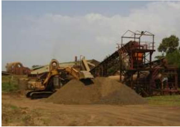
Plant crushing and screening operations located on Mining License ML 4651
