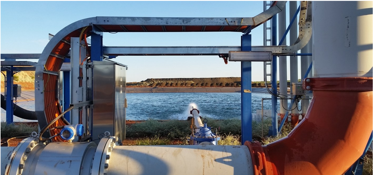
Figure 1: Water from wet commissioning activity is returned to the process ponds - stockpiles of high-grade crushed native copper ore in background will be the first ore to be processed.
