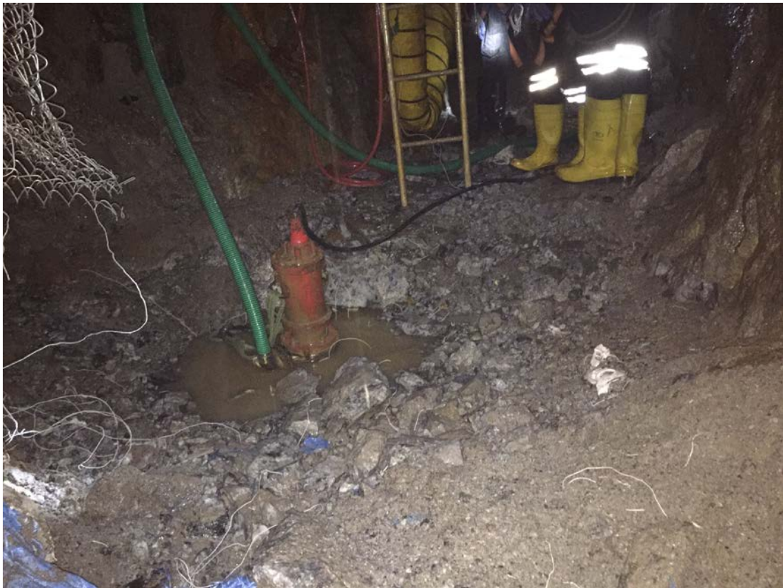
Figure 8: Initial Blast to deepen Pandeniya main shaft to 45m
