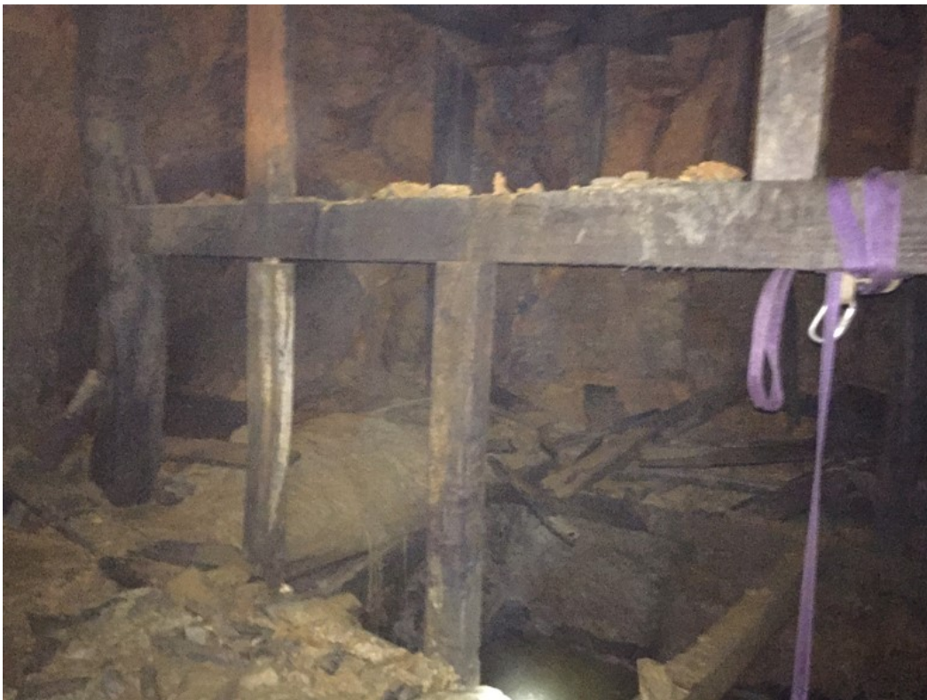
Figure 6: South Winze and lower Historical workings
