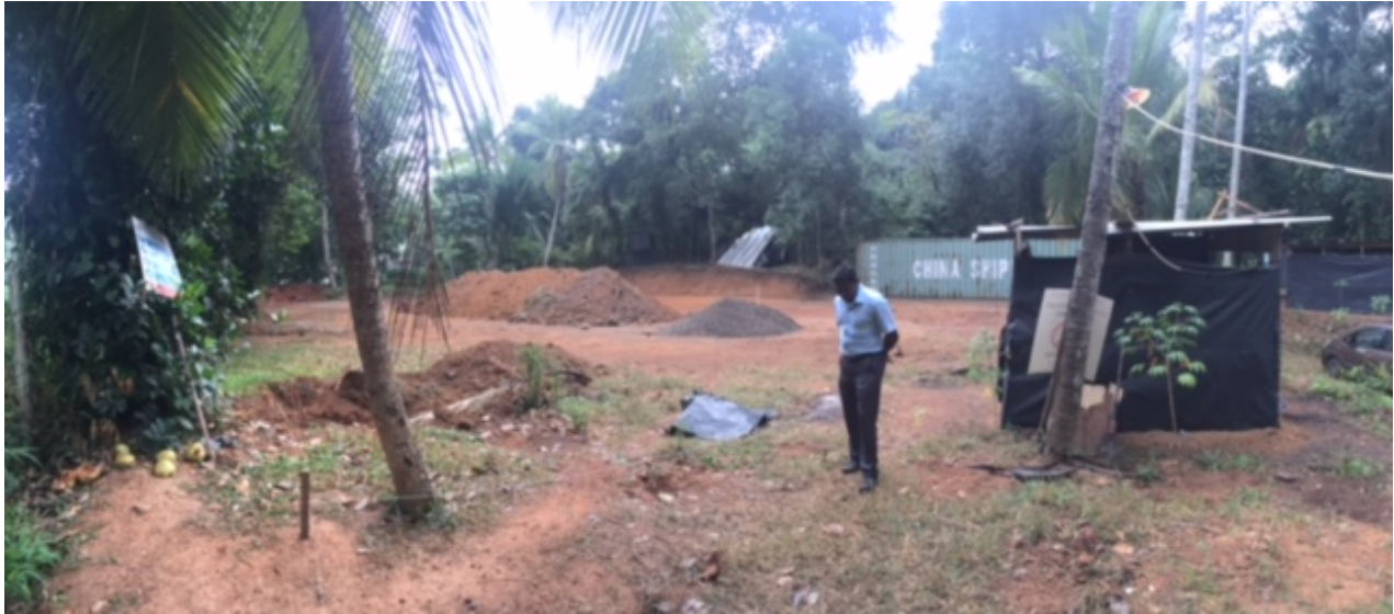
Figure 9: Site works commencing at the Warakapola hub
