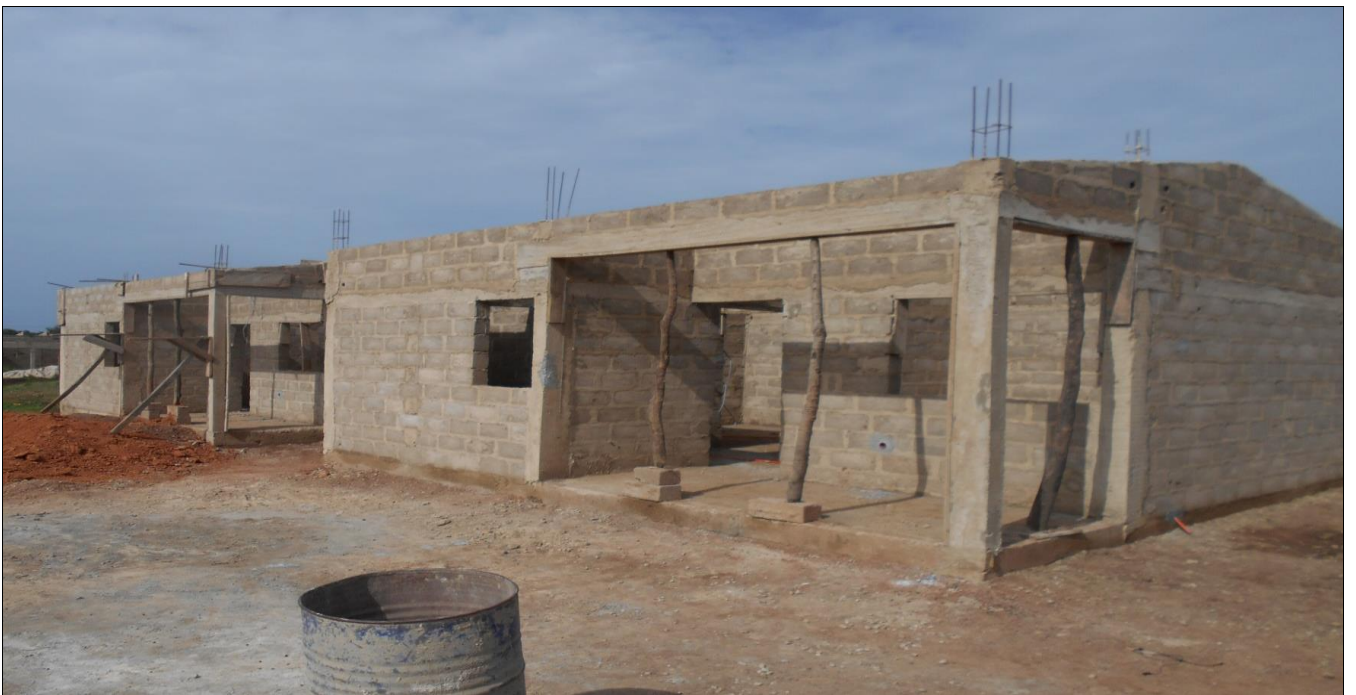
Construction of last of 18 relocation houses
