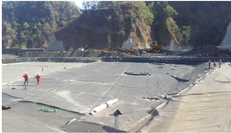
Image 5 – Lining of Cell 6 on the KKV Heap leach pad
