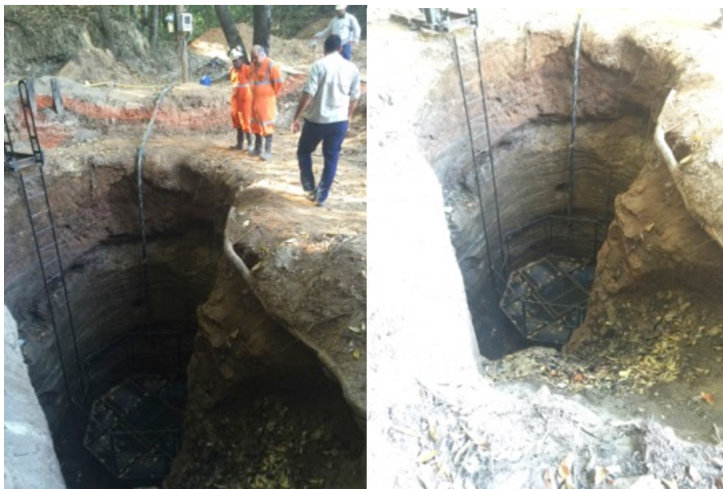
Figure 2. The existing Cuca shaft, with a depth of 18m, is being dewatered and made safe prior to further bulk sampling.
