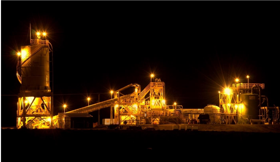
Olaroz liming plant at night
