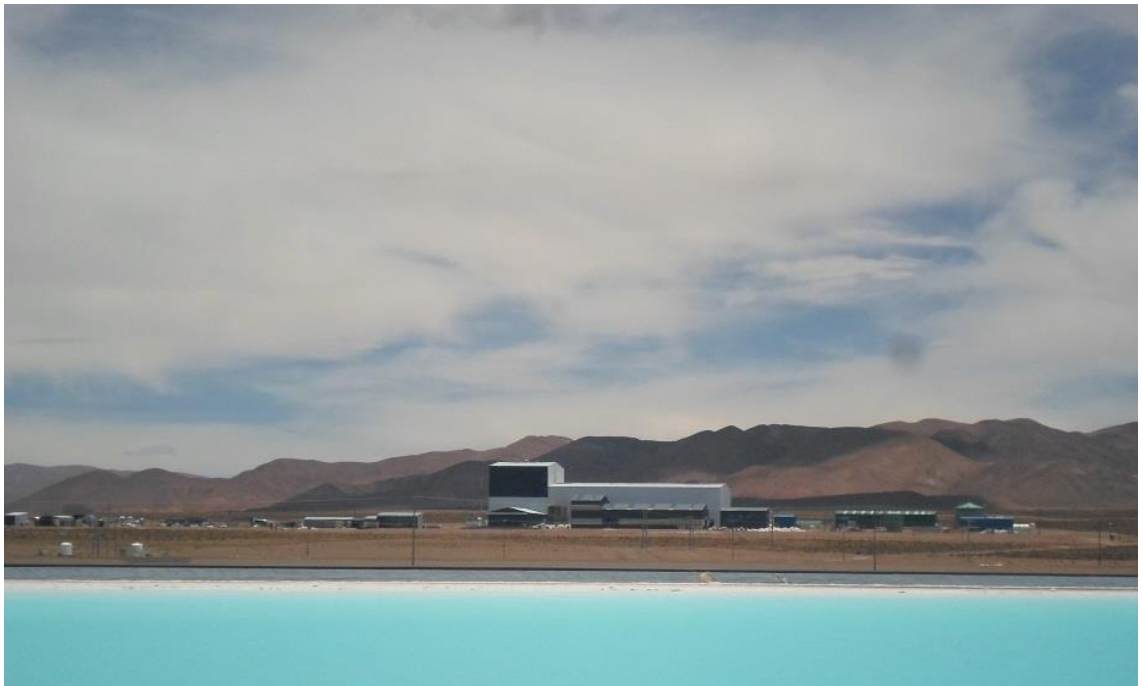
Olaroz Lithium Facility
