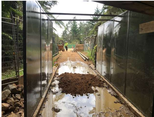
Figure 3 - View from the portal during installation of the air lock structure
