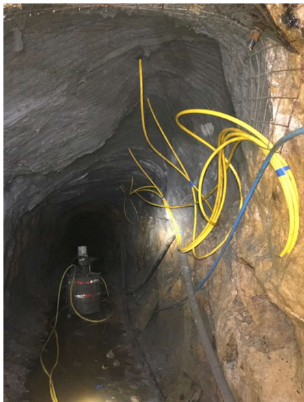
Figure 2 - Shotcreting to seal a historic orepass
