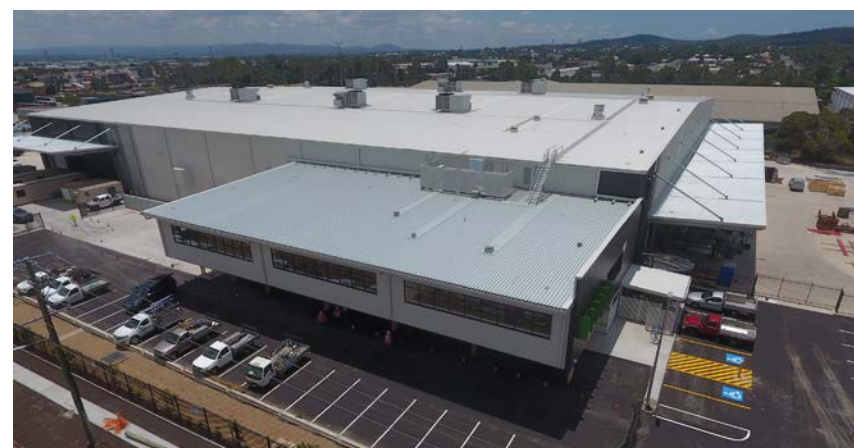
Construction progress: new Brisbane wholesale facility
