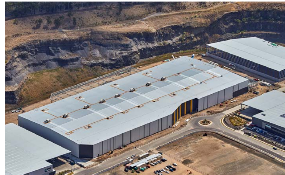
Construction progress: new Sydney Contract Logistics facility.
