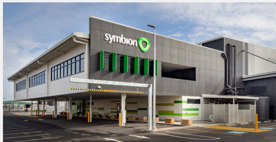
New Brisbane wholesale distribution facility
