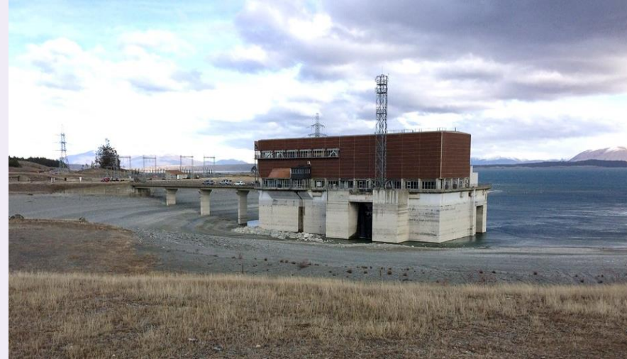
Genesis Energy's Tekapo B power station
