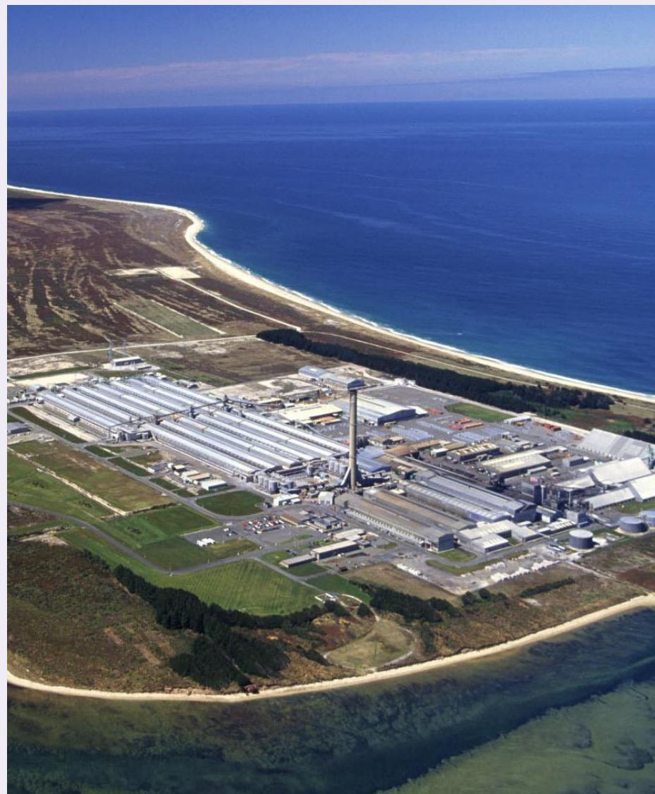
New Zealand Aluminium Smelter, Tiwai Point
