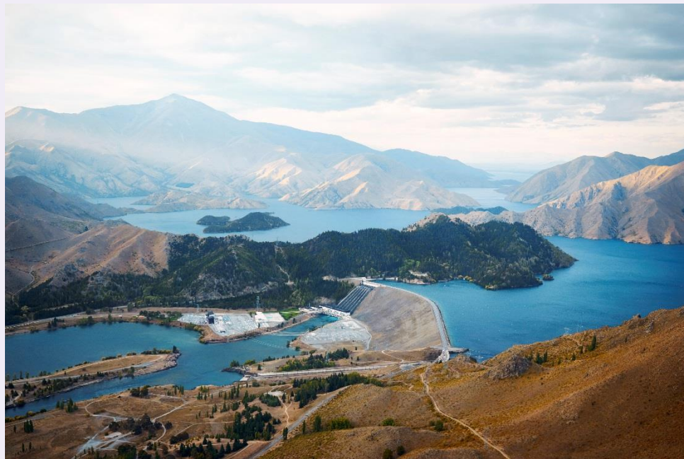
Meridian Energy's Benmore power station
