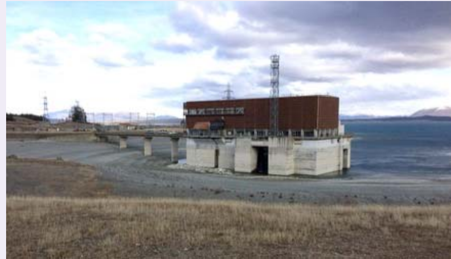
Genesis Energy's Tekapo B power station
