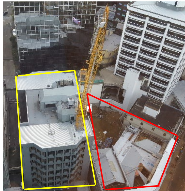
8-14 Willis Street (yellow) and Stewart Dawsons Corner (red).
