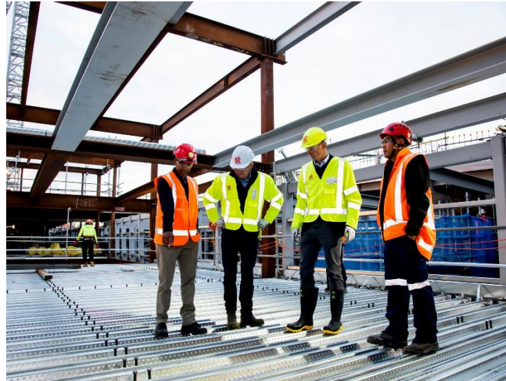
Installation of Comflor in Westfield development in Newmarket, Auckland
