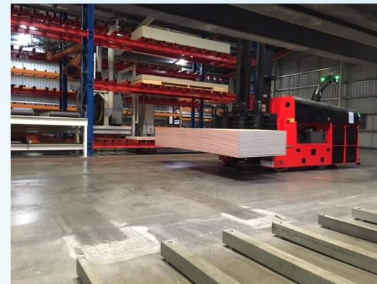
Plasterboard Handling & AGV Systems
