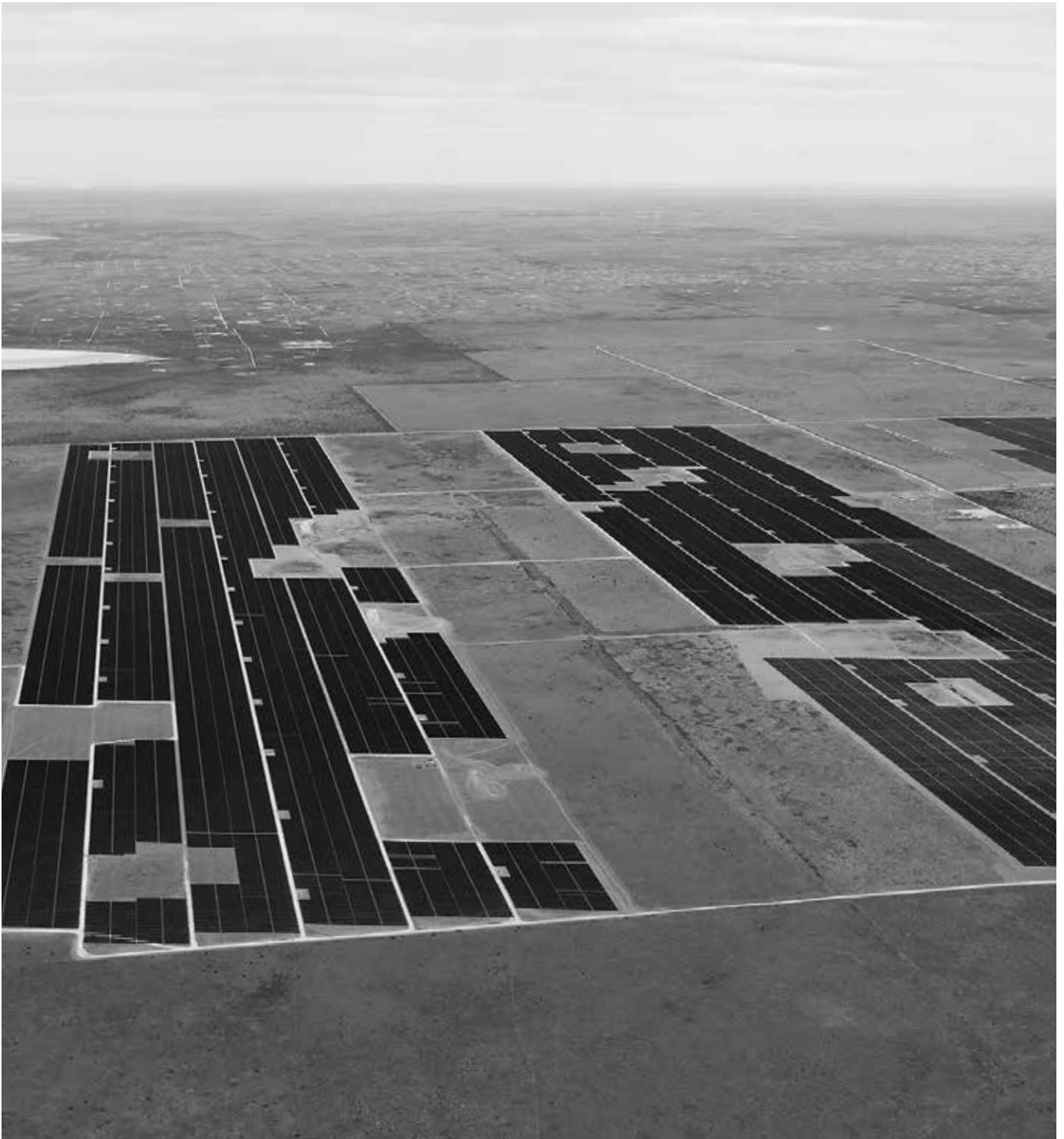
Prospero Solar project, Texas, USA.
