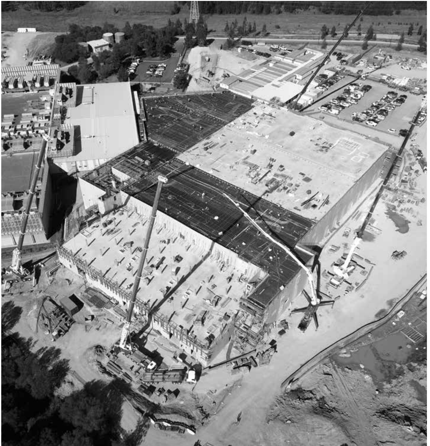
Construction continues on CDC's Eastern Creek 3 data centre, Sydney.
