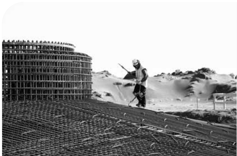
Above & right: Waipipi Wind Farm project team constructing wind turbine foundations.
