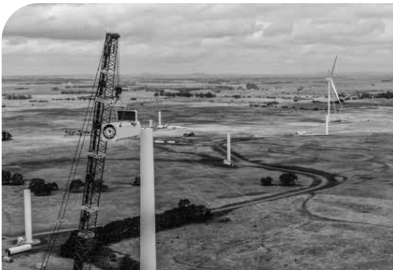
Left: Wind turbine nacelle lift and fitting. Below: Foundation pour.
