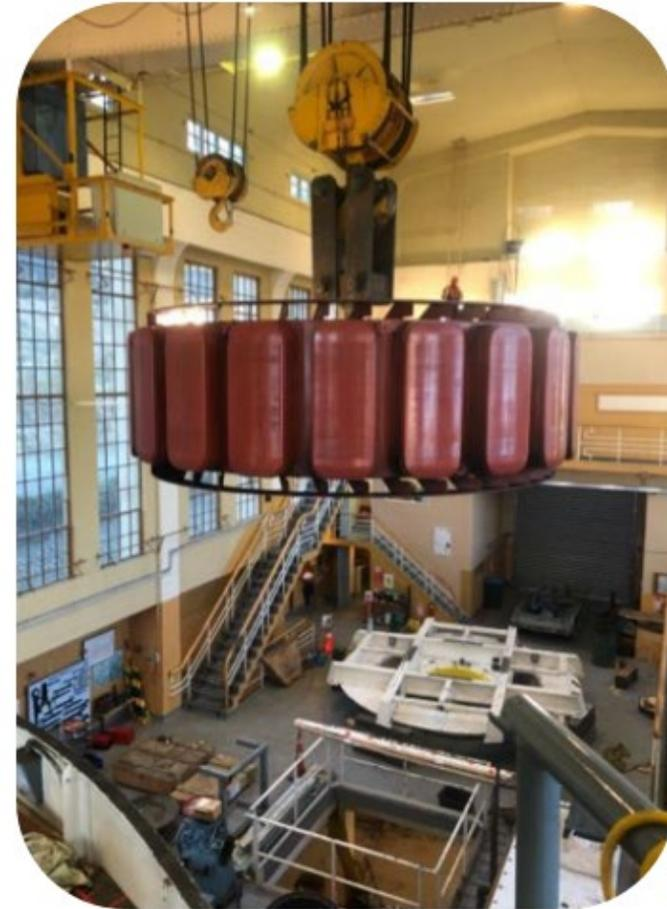
Highbank rotor being lifted into the stator
