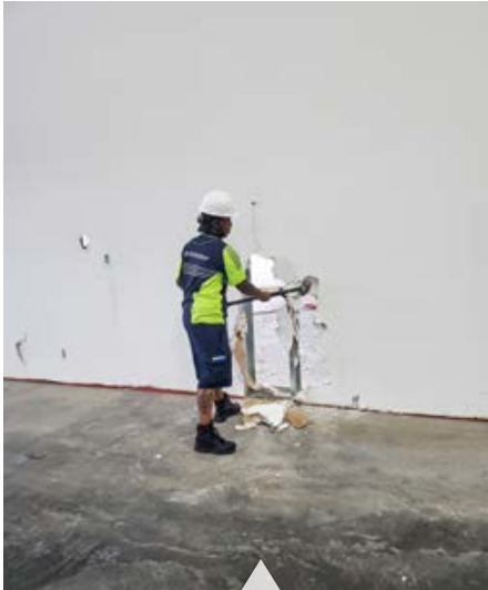
Devyne Gilliam removing the wall in the Atlanta warehouse
