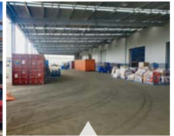
After addition of canopy
