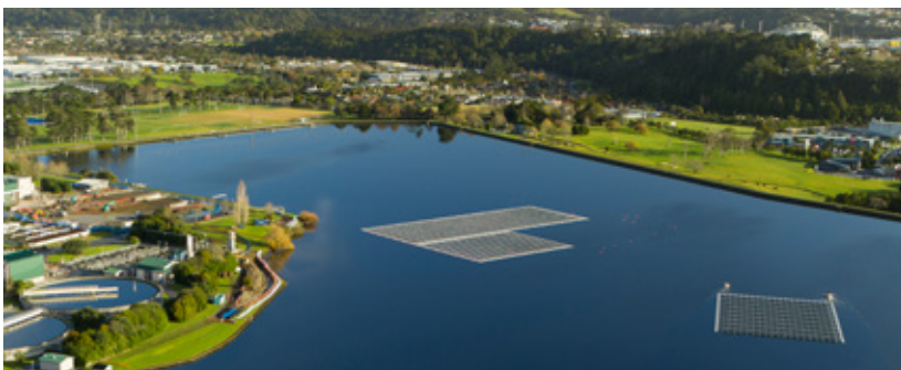
New Zealand's first floating solar farm, built by Vector Powersmart for Watercare, produces the same amount of electricity as would be needed to power approximately 10,000 homes
