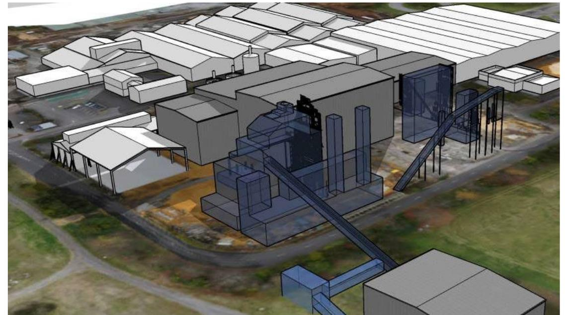
*Grey and translucent blue indicates new plant and equipment to be built beside existing end-of-life plant which will be decommissioned on completion*
