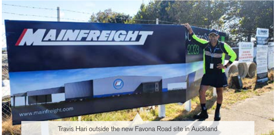
Clearing the site.
