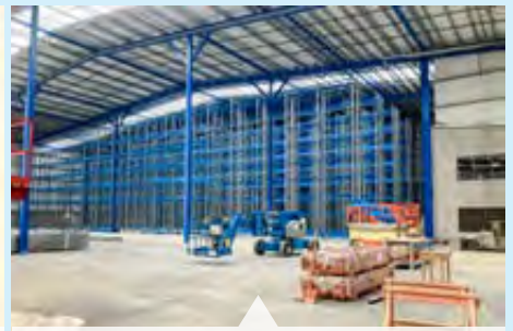
New racking being installed (15,000 pallets)
