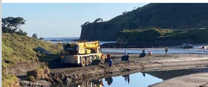
The sand beach that the crane and 7 truckloads had to cross
