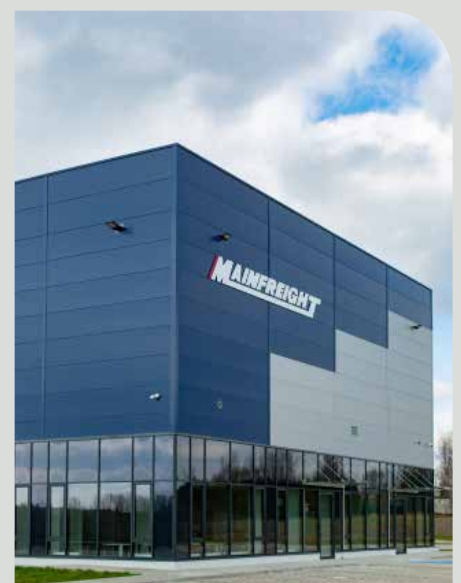
Our new Cross-Dock Facility in Katowice, Poland
