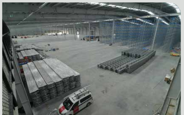
Racking installation underway...55,000 pallet spaces
