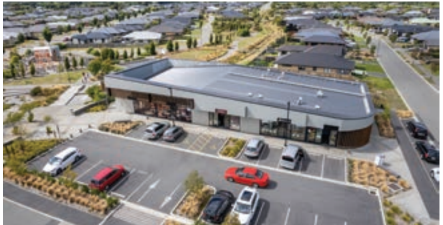
Stonebrook Retail Centre, Rolleston, Selwyn, Canterbury
