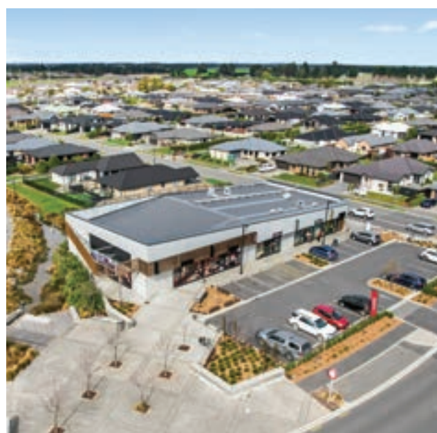
Stonebrook Retail Centre, Rolleston, Selwyn, Canterbury
