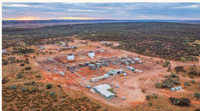
Mereenie plant located in the Amadeus Basin, Northern Territory, Australia.
